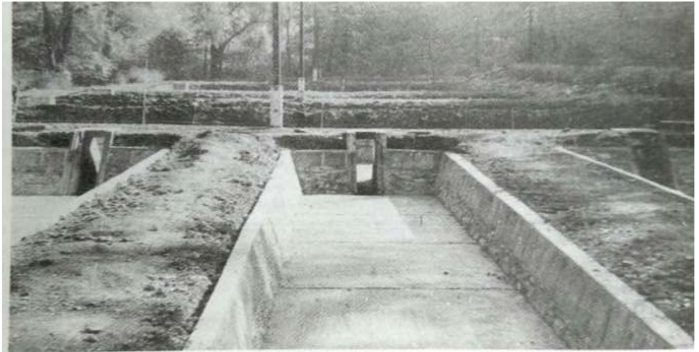
A raceway farm under construction. (Courtesy of J. Kovari.)
