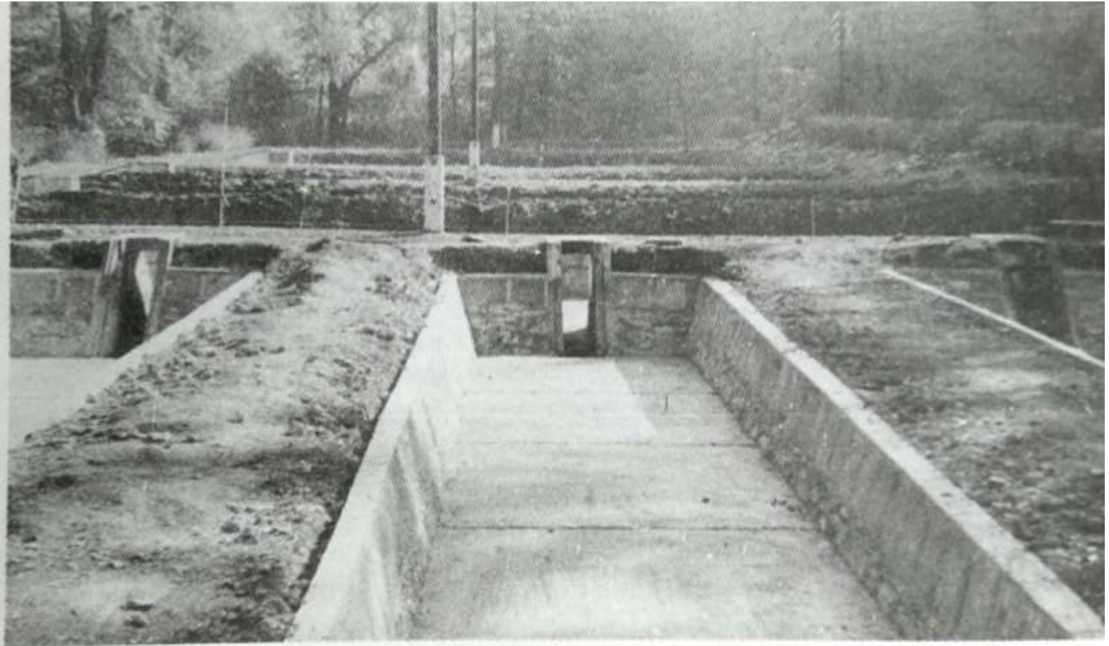
A raceway farm under construction. (Courtesy of J. Kovari.)
