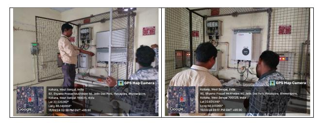
As per resolution of the above mentioned meeting, Asutosh College Solar plant Committee has replaced 10 KVA String Inverter (**Make** – Power-One Micro Systems Pvt Ltd) at existing 10kWp SPV Power Plant System installed at Ashutosh College.
